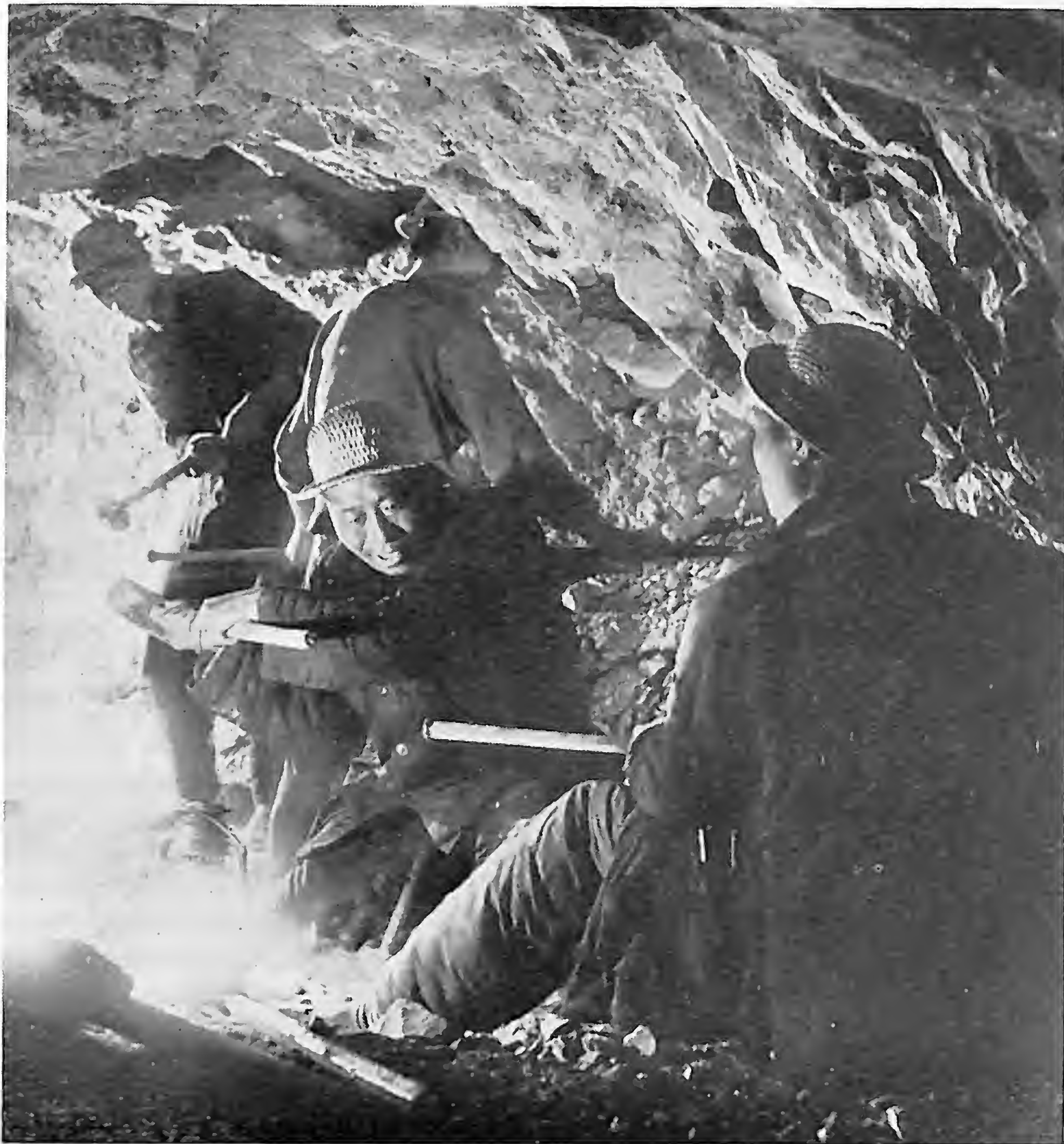
Inside Dawn Tunnel.
